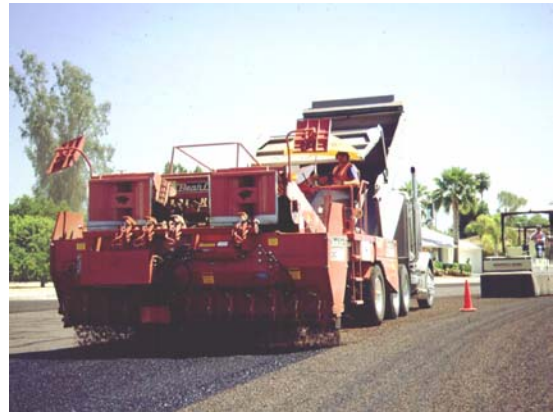
Figure 4-3: Spreading Precoated Aggregates
