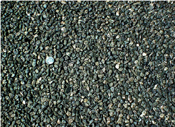
Figure 4-6: Finished Chip Seal Before Applying Fog Seal and Sand
