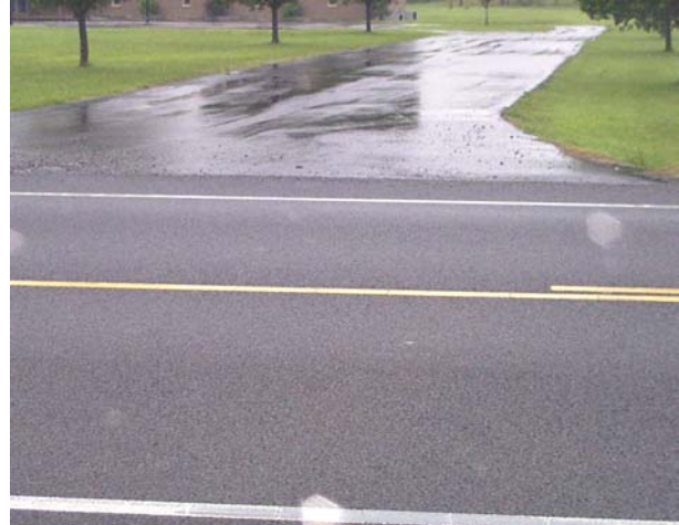
Figure 2-4: Free-Draining RAC-O Next To DGAC
