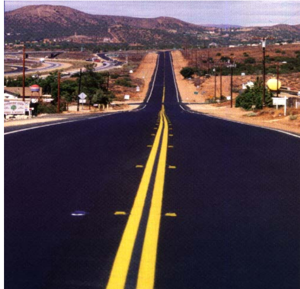
Figure 2-3: Finished RAC-G Pavement
