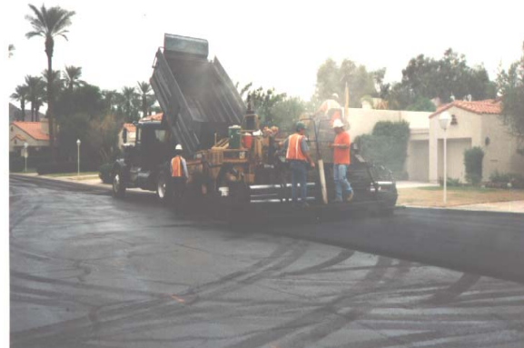
Figure 4-1: Unloading RAC-G Into Paver Hopper
