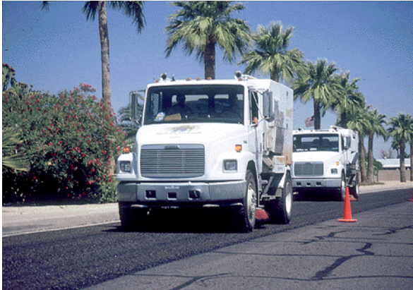
Figure 4-5: Sweeping Chip Seal To Remove Loose Cover Aggregate
