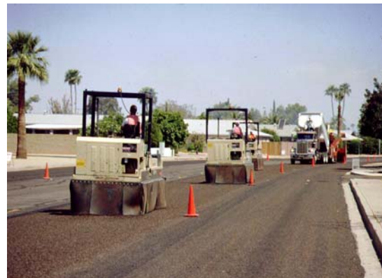
Figure 4-4: Rubber-Tired Rollers With Skirts On Chip Seal
